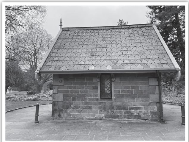
Old Magnesia Well Pump Room
